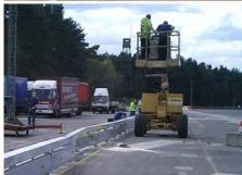
BikeGuard, an award winning system, is fully tested to BS EN 1317 part 2 and fully approved by the Highways Agency for use on the UK trunk road network. ("HA Accepted EN1317 Compliant Road Restraint Systems" - Miscellaneous Section). BikeGuard is a high quality, lower steel beam that can be attached to "W" beam type safety barriers and Open Box Beam systems to improve the safety performance of these barriers when impacted by motorcyclists.
