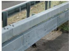
Used extensively throughout the UK, BikeGuard prevents motor cycles and particularly their riders from sliding under the barrier and becoming snagged on the barrier support posts. This considerably reduces the extent of motorcyclist injuries and is a product endorsed by both coroners and emergency services.
