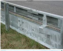
BikeGuard is manufactured in galvanised steel, and is fixed to the barrier with specially shaped brackets which attach to the rear of the barrier rail, allowing the BikeGuard to perform independently of the barrier during impact. The BikeGuard system utilises slotted holes and a hanging bracket to enable horizontal and vertical adjustment. The brackets are secured to the back of the barrier with purpose designed fixings to suit different barrier types.
