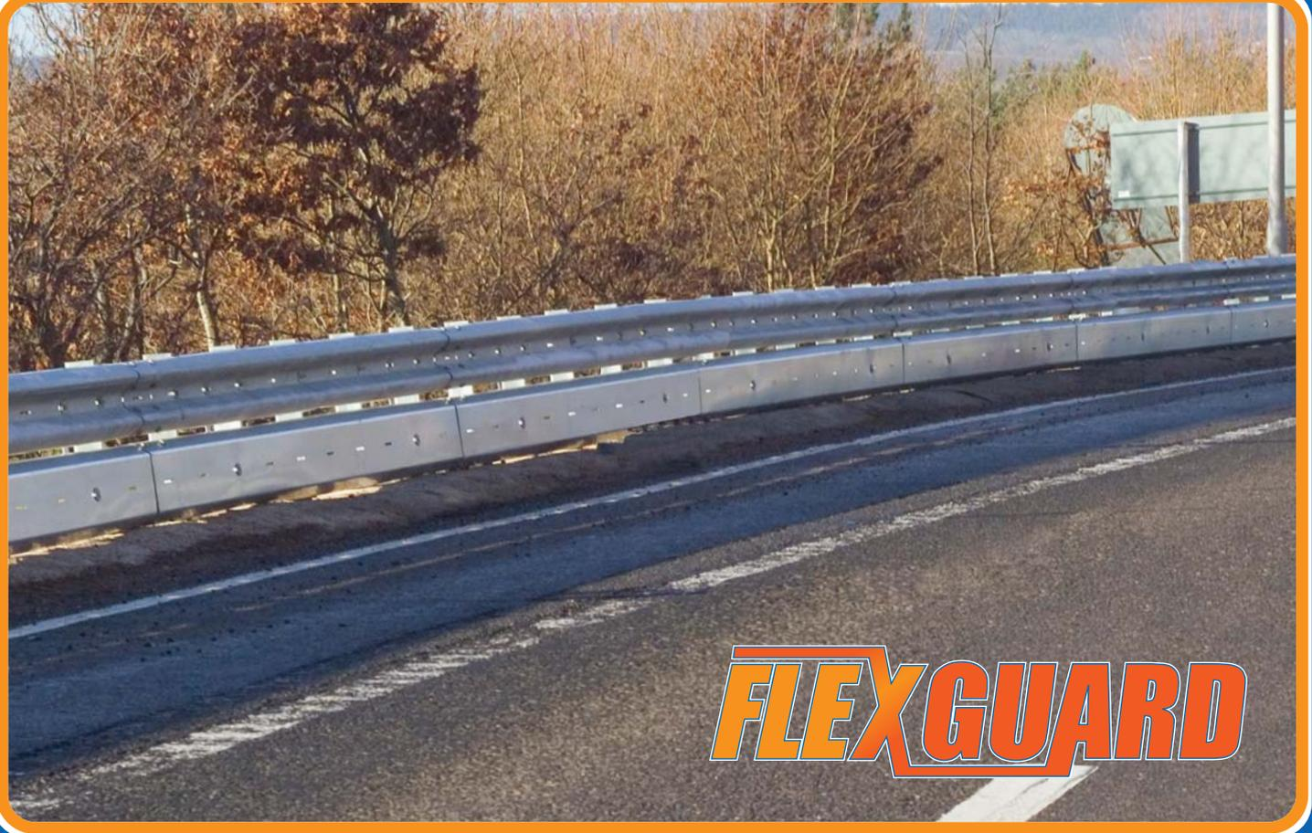
FLEXGUARD is a single sided retro fitted barrier system designed to protect motorcycles from travelling beneath road side barriers.
