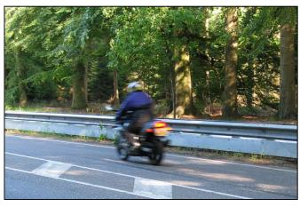
It is widely accepted that the risk of (fatal) injuries to motorcyclists can be easily and significantly reduced by covering the supporting posts of the crash barrier.
