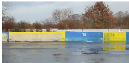
Transition from precast Delta-bloc to in-situ cast STEP H2 – W4 - C
