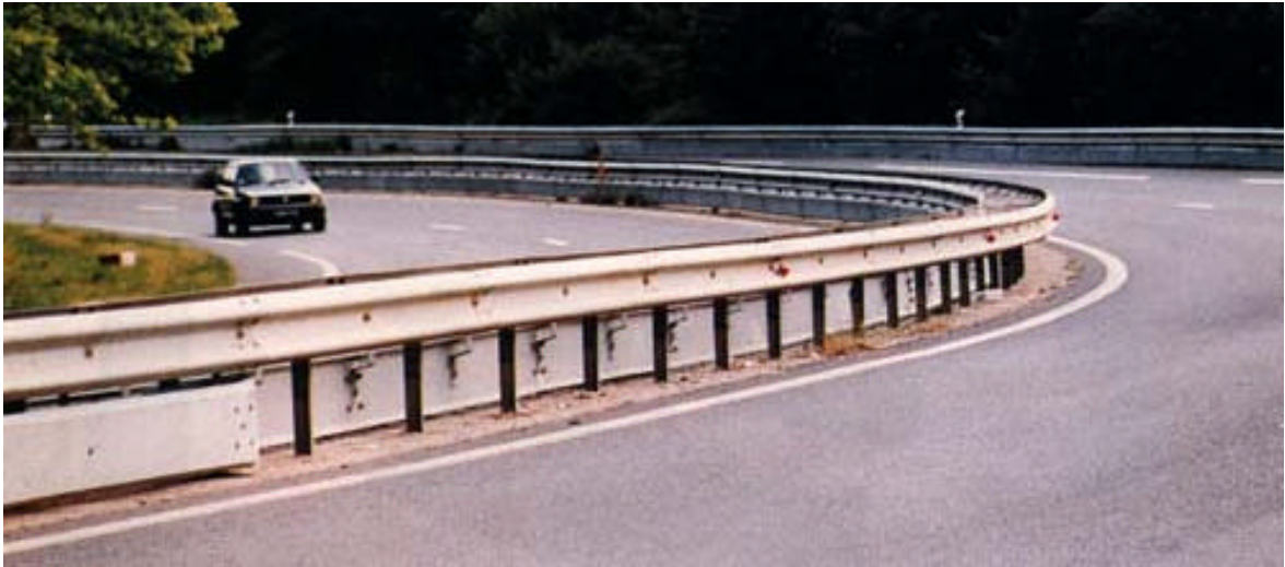
Figure 3: Photograph of the ‘Ecran Motard’ fitted to an existing guardrail.
