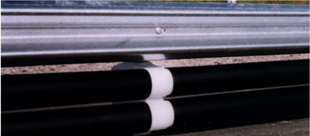
Figure 9: Photograph of “Mototub” fitted to existing barrier system.
