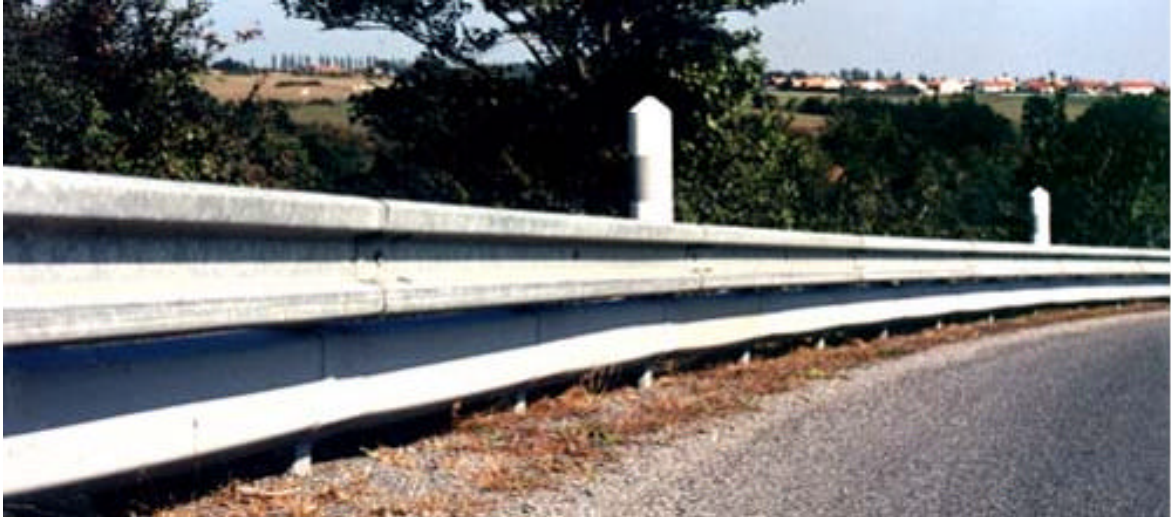
Figure 5: Photograph of the “Plasti-rail” fitted to existing barrier system.
