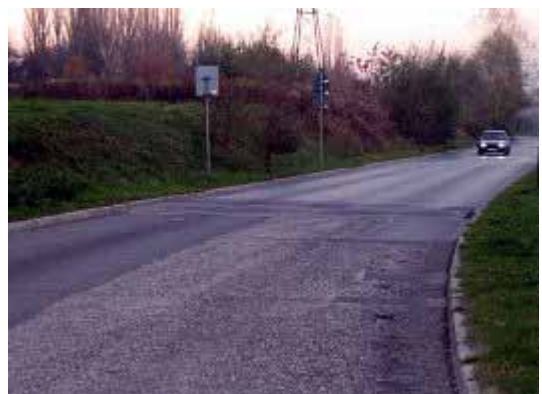
Figure 6 Speed bumps with low visibility and in a curve.(source: id.)
