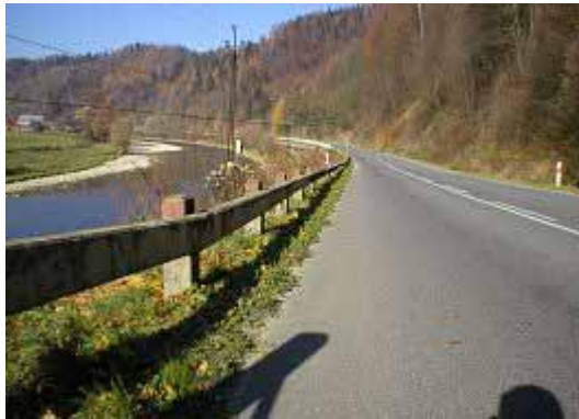
Figure 4 Road barriers: concrete barrier (Zakopiańska) and steel barrier. (source: ITC, Bulgaria and the Cracow University of Technology)
