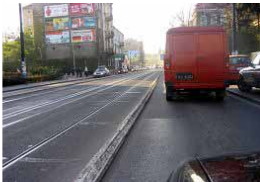
Figure 5 Kerb as a lane separator (width of the lane is 3,50m), (source: id.)
