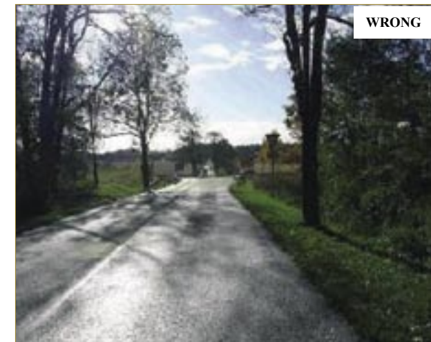
Figure 9: Intersection not visible 125 m ahead: unexpected braking and high speed cause rear end collisions [16]
