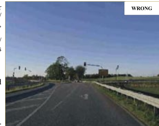
Figure 5: Junction, perceptible only at 100 m distance: the minor road seems to be the main road, unexpected braking and high speed at this point cause rear end and sideswipe collisions [16]
