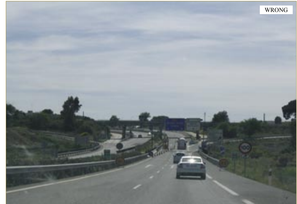
Figure 45: Two critical points: maintenance point and an exit road without transition and/or moderation (150 m ahead). [22]
