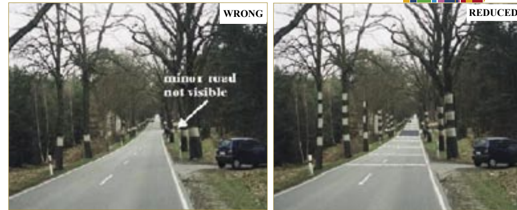
Figure 6: Minor road not visible early enough: unexpected braking and high speed at this point cause rear end collisions [21]
