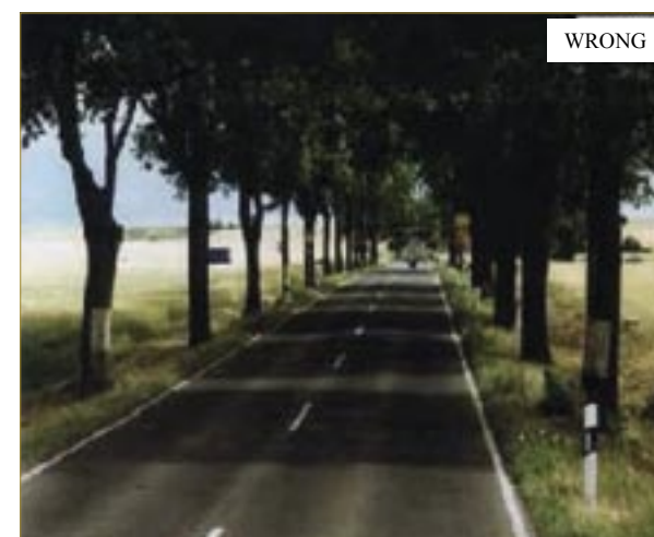
Figure 43: Sudden change of road characteristic: new crossing is not instructed by moderated transition area (150 m ahead). [16]
