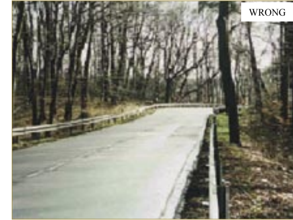
Figure 48: How many traffic signs you can detect? Non visible course at a dangerous accident bend [20]
