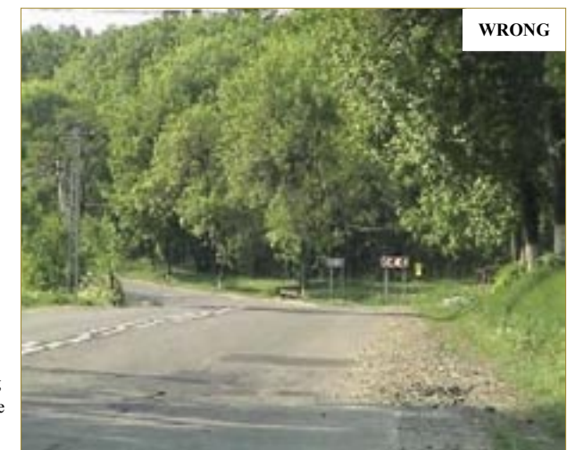
Figure 8: Course of the bend is not perceptible because inside bend is obscured: unexpected braking, steering manoeuvres and high speed cause drive off the road [23]
