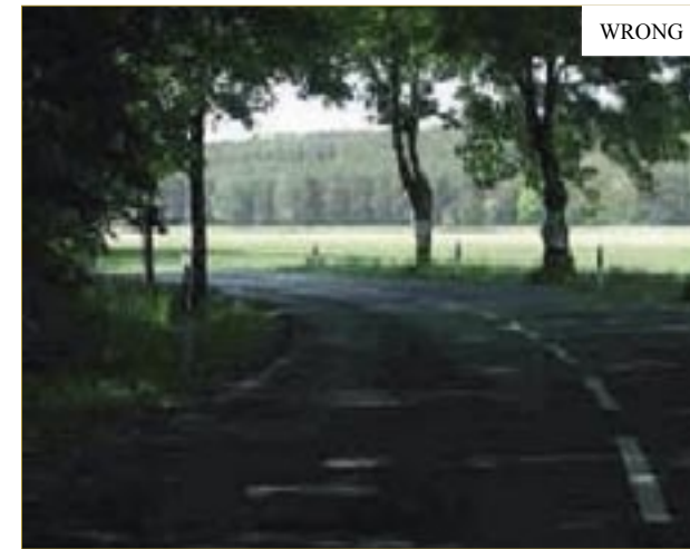
Figure 13: Tendency towards the outside bend by misleading gaps in the framing, obstructed inside bend [22]
