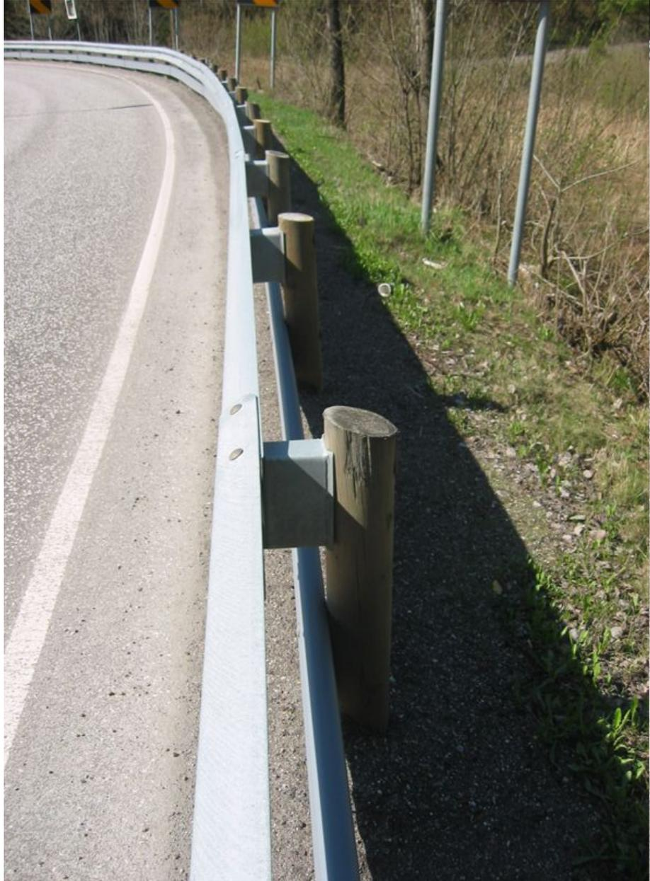
New guardrail design protects sub-rail against impact of snow plough
